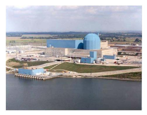
Liquid effluents from the Clinton station are permitted to be released into the eastern arm of Clinton Lake, a 4,900-acre man-made cooling lake, in accordance to release limits governed by the station's license with the NRC and the station's IEPA NPDES permit. The outflow from Clinton Lake falls into Salt Creek, a tributary of the Sangamon River. No liquid effluents were discharged in 2021.
