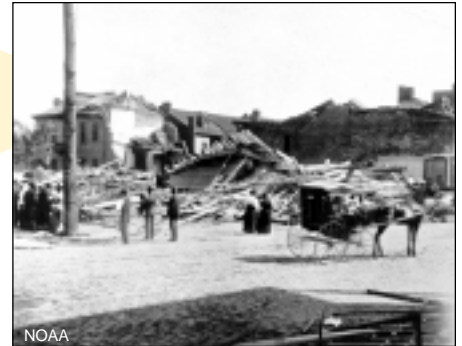
St. Louis tornado damage, May 27, 1896.
