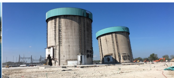
Zion Station in October 2018
