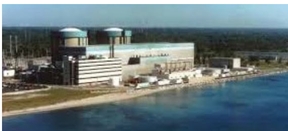
Zion Station prior to decommissioning
